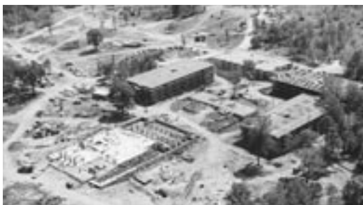
▲ The Jonsson campus under construction
