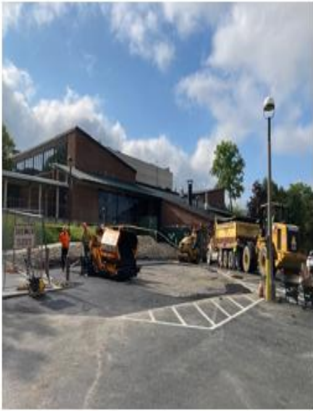
New ADA Compliant ramp being installed outside of Dining Hall
