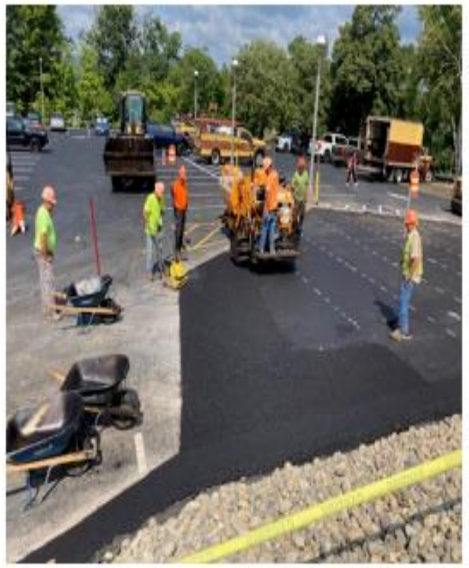
New ADA Compliant ramp being installed outside of Dining Hall
