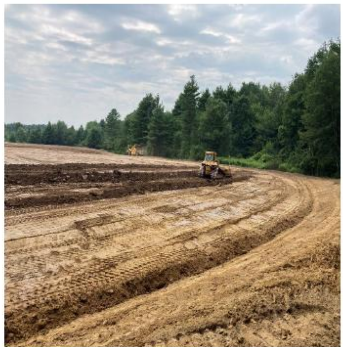
Working on new baseball field site
