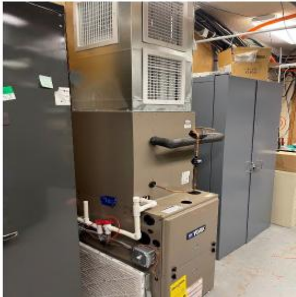
New AC unit installed
