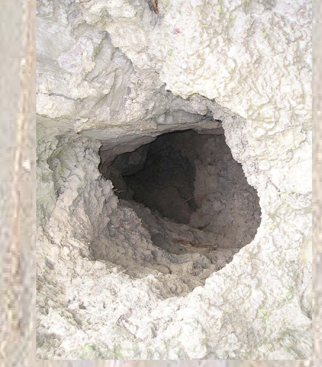
Intact pipe outlet on hillslope
